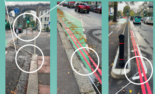
Overlapping elements create a messy effect. White hash markings are unnecessary clutter, green lane paint should begin further from kerb to avoid red line overlapping.
